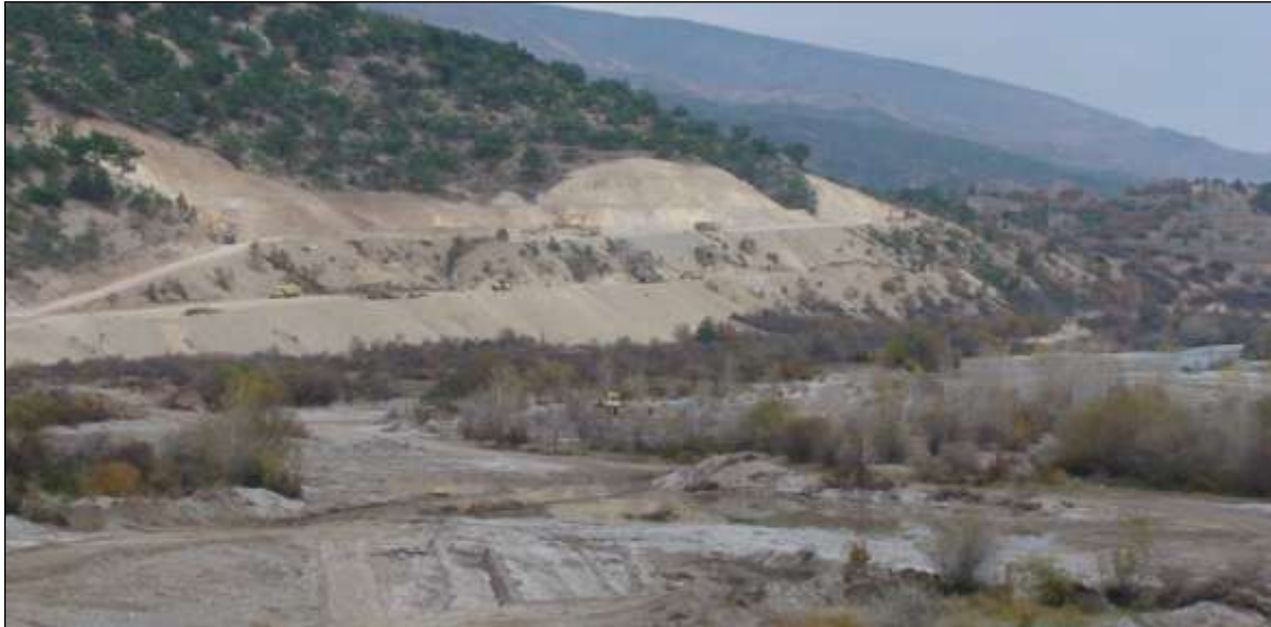
Figure 2. Reşadiye-I HEPP Project site
