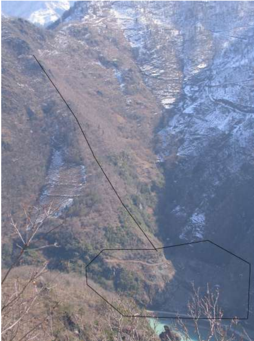
Figure 2. ARALIK HEPP Penstock and Powerhouse Location
