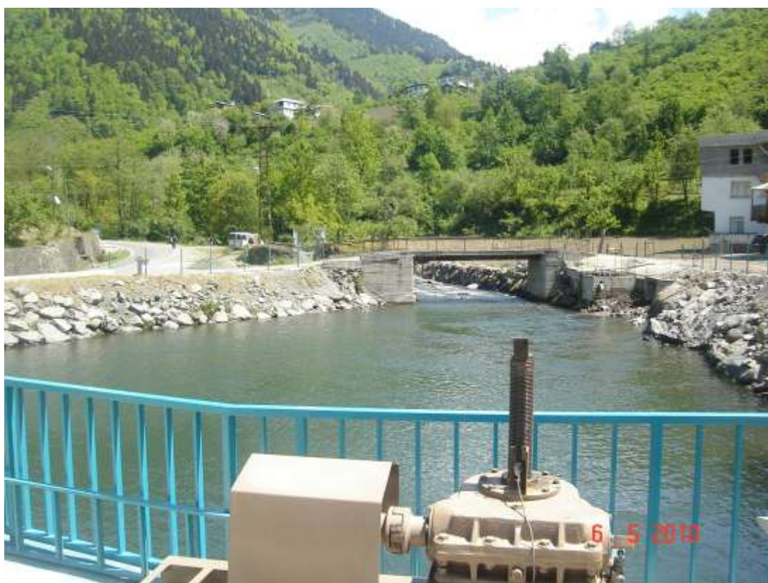
Figure 5. View of reservoir from weir body.
