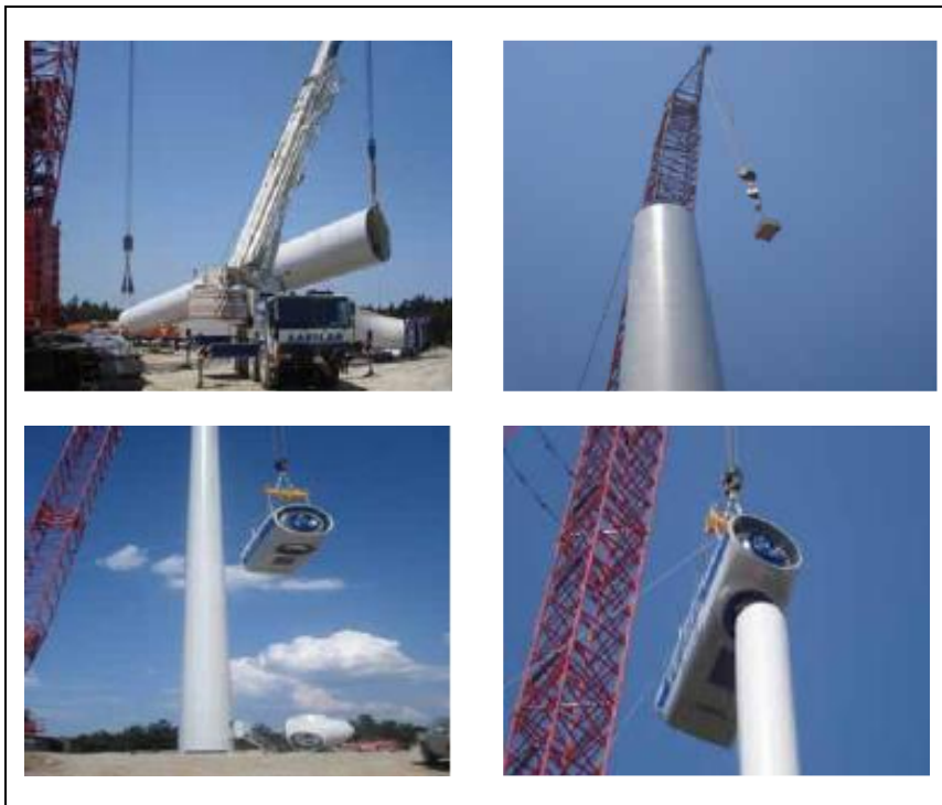
Figure 1 Pictures from the Bandırma WPP site during installation of turbines, July 2009
